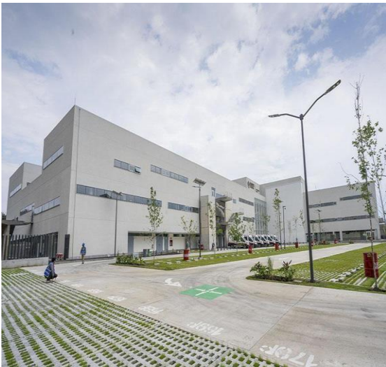
Hospital General Tláhuac
